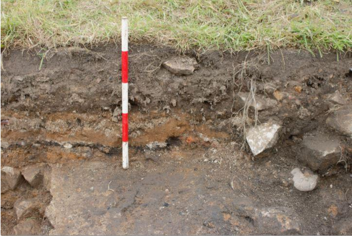
Plate 3: South-east facing section off Trench 1 showing the cut (Context No. 106) filled with the demolition rubble (Context No. 102).
