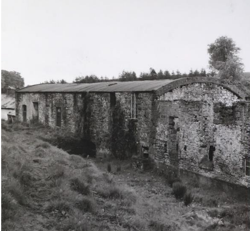
Figure 2: Photograph of the rear of the structure prior to its demolition (possibly 1970s). this picture illustrates the terrace cut into the slope to accommodate the mill structure (image provided by Keith Beattie LNLP).
