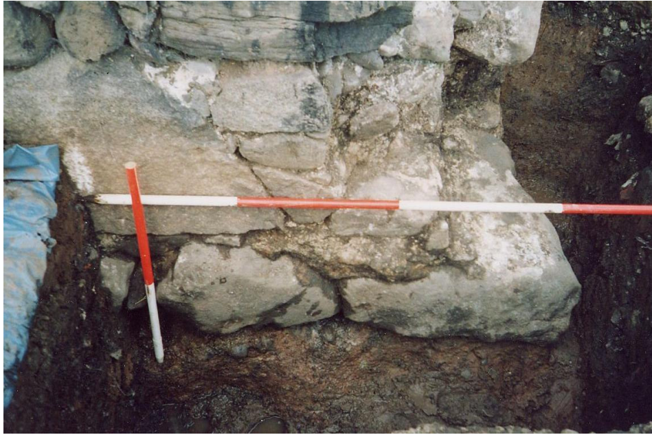
Plate 3: Exposed length of south-facing wall
