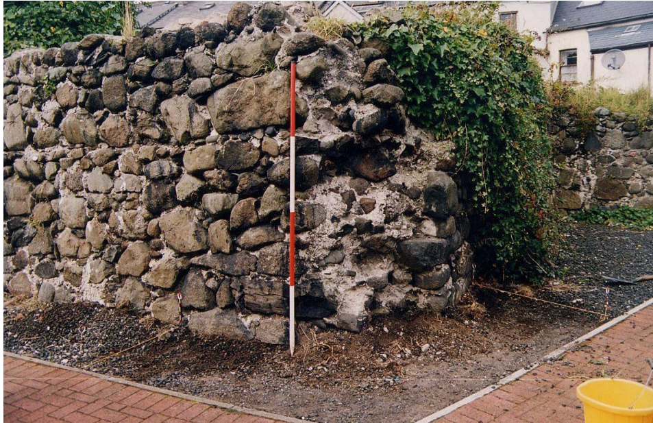
Plate 1: General view of corner before excavation
