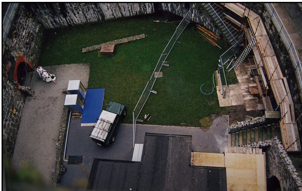
Plate 1: View of the magazine and inner ward from the roof of the keep.
