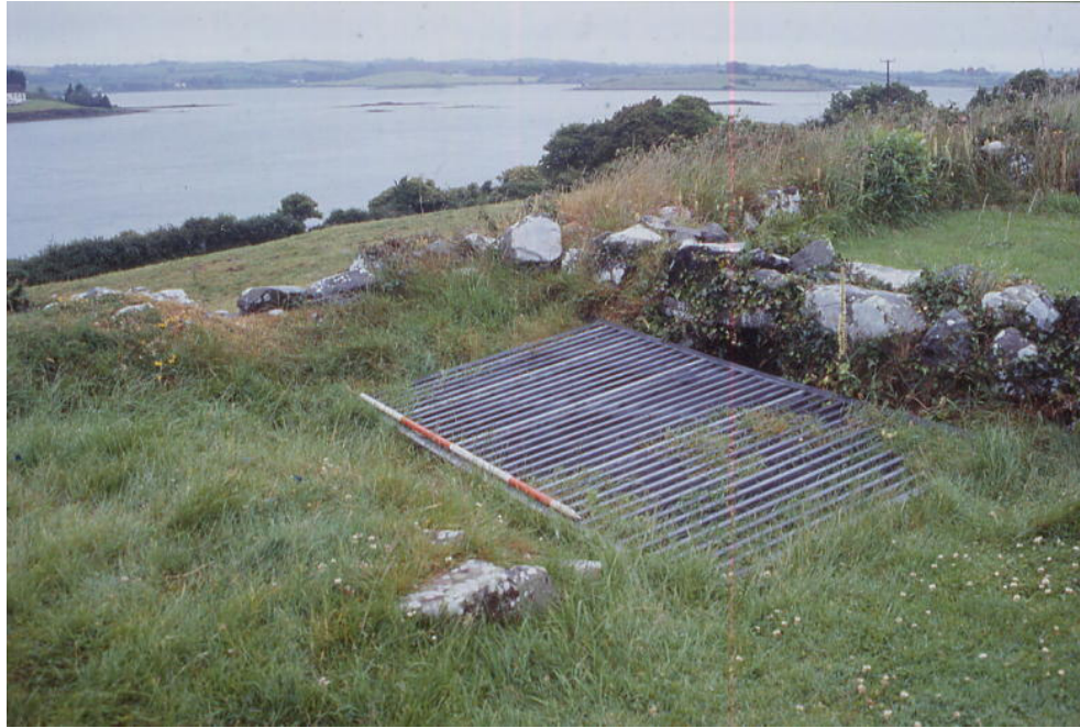
Plate One: The exposed pit prior to the removal of the old safety grill looking west.
