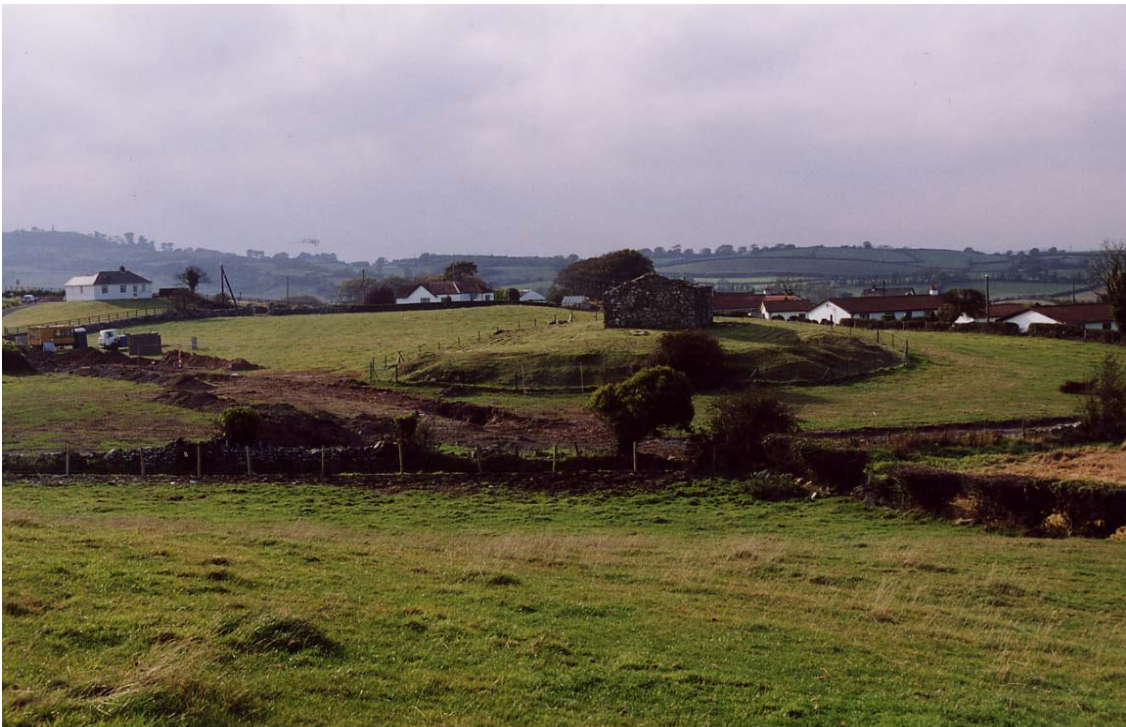
Plate 6: Church and Water Service pipe trench with trenches visible, looking west
