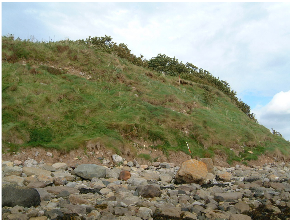
Plate Fifteen: The actively eroding southern cliff of the main island (looking northeast)
