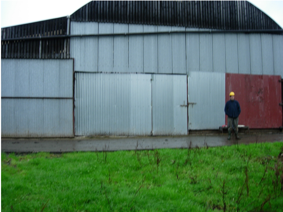
Plate One: General view of site, looking south-west
