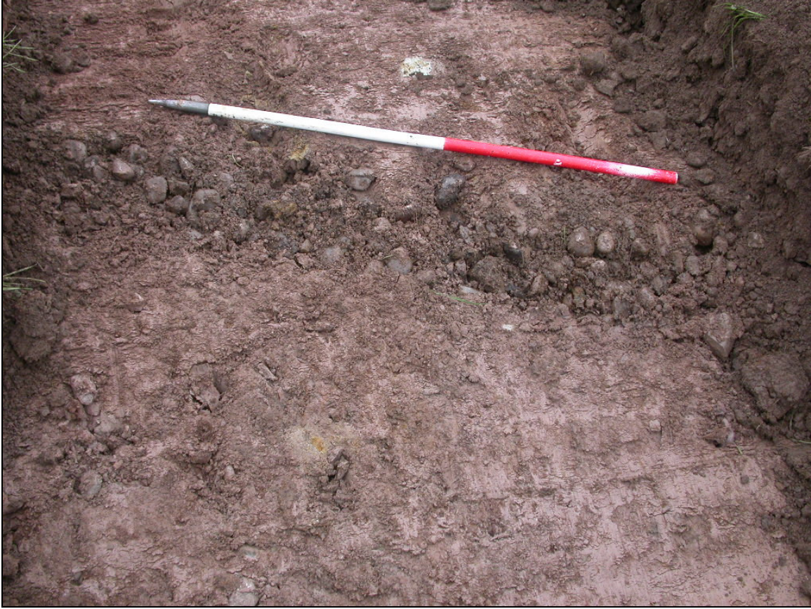
Plate 4: 3" drainage pipe in Trench 2 protected by gravel covering.
