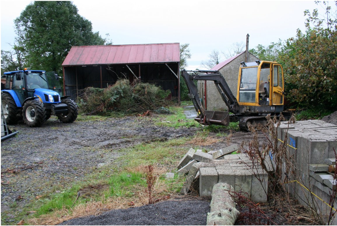
Plate 1 General shot of development site showing the hard packed gravel surface.
