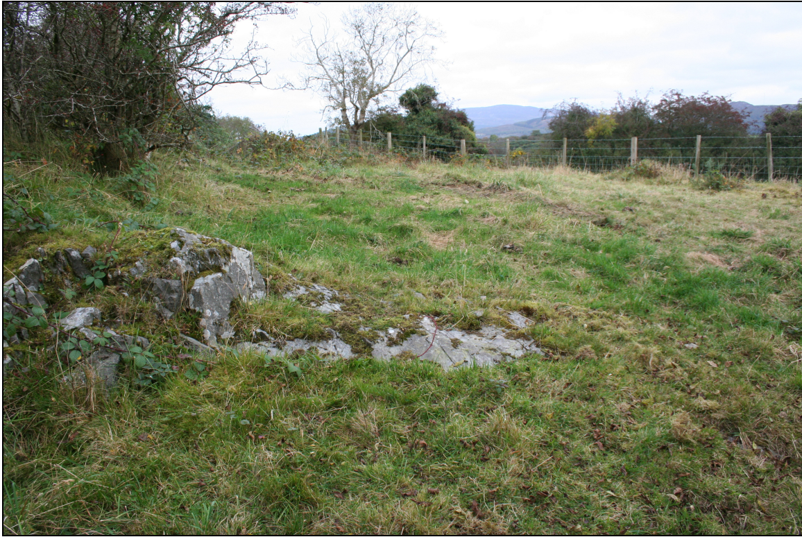
Plate 7 General shot, looking NE, showing the proposed access way to the development site and the frequent bedrock outcropping of the area.
