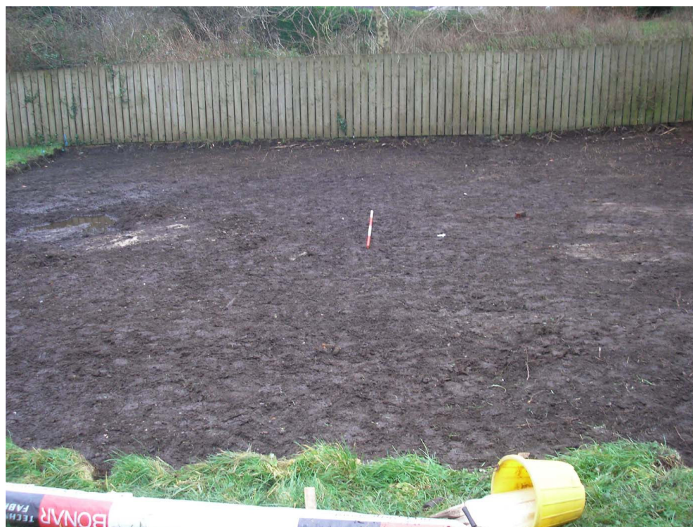
Plate 11: Application area following excavation to a depth of 0.3m, looking south.
