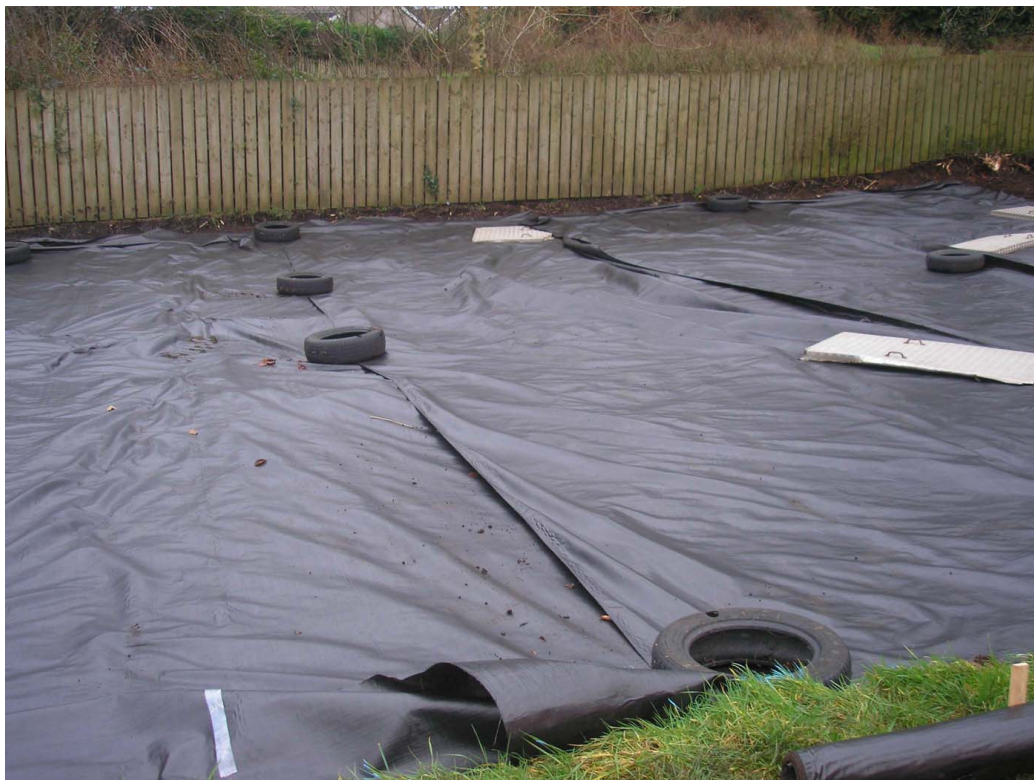
Plate 12: Application area showing the layer of Geo-textile, looking south.
