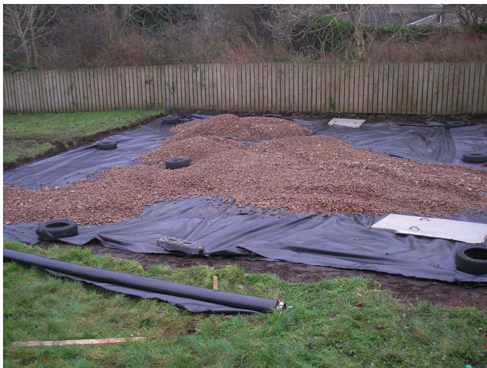
Plate 13: Application area showing gravel hardcore being laid down, looking south-east.
