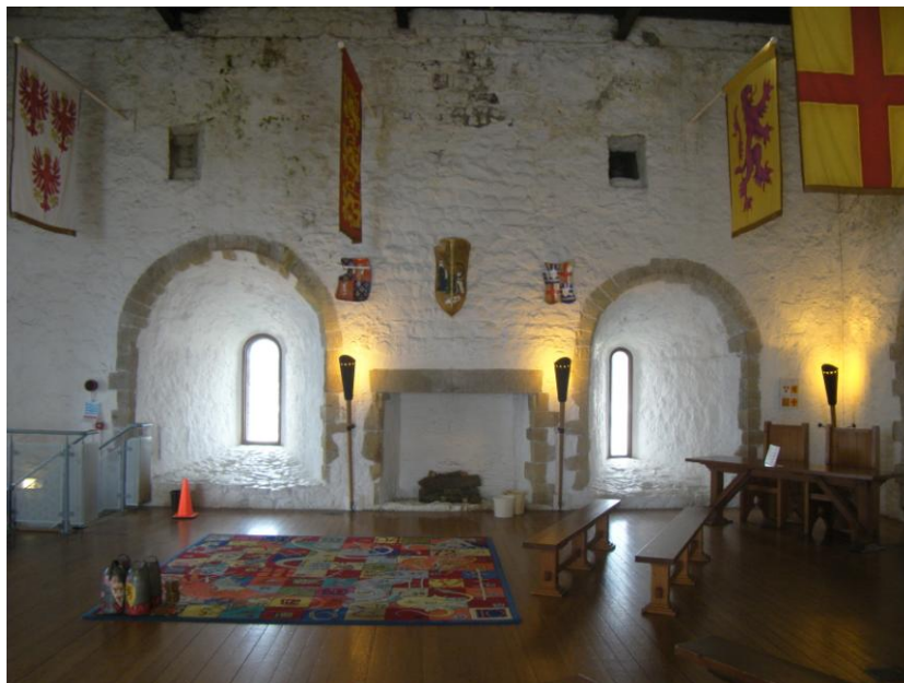
Plate 18: View of third floor fireplace, looking west
