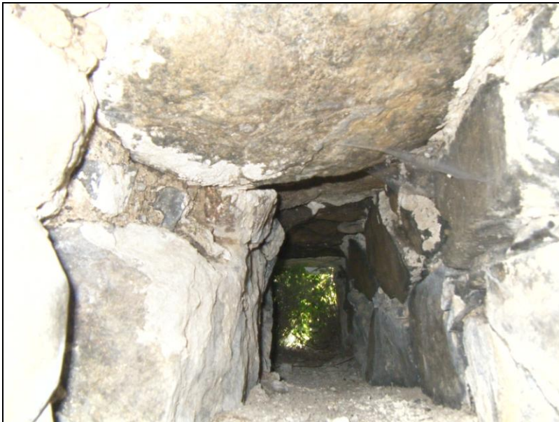
Plate 08: View of interior of weephole C232, looking west
