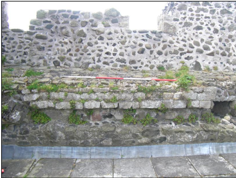
Plate 01: Pre-excitation view of Trench 1 at southern wall-walk, looking south [scale 2m]
