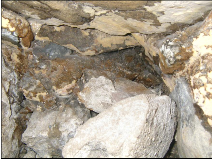
Plate 09: View of interior of weephole C232, looking east
