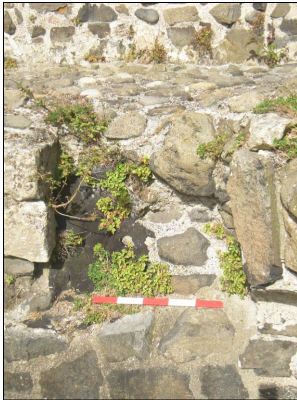
Plate 10: Trench 3, pre-excavation view, looking west [scale 0.5m]
