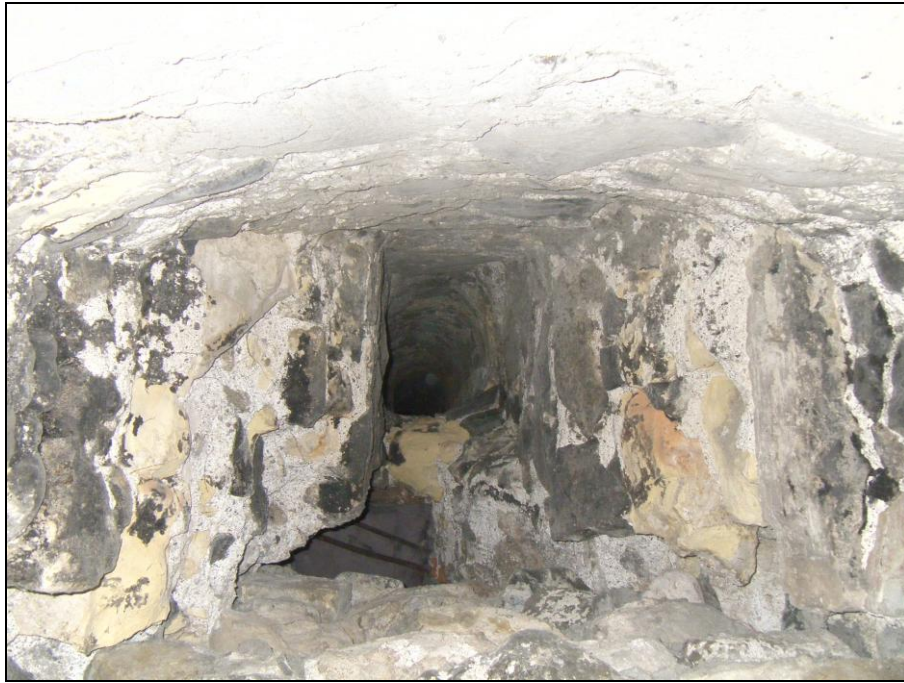
Plate 19: View up chimney flue from second floor fireplace
