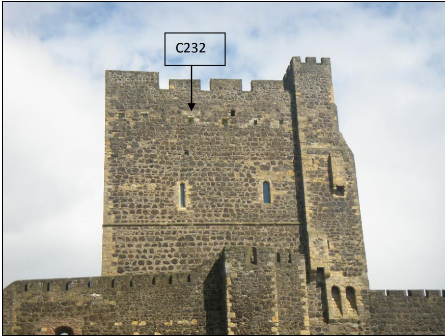
Plate 07: West wall of Keep, weephole C232 and other weepholes, looking east
