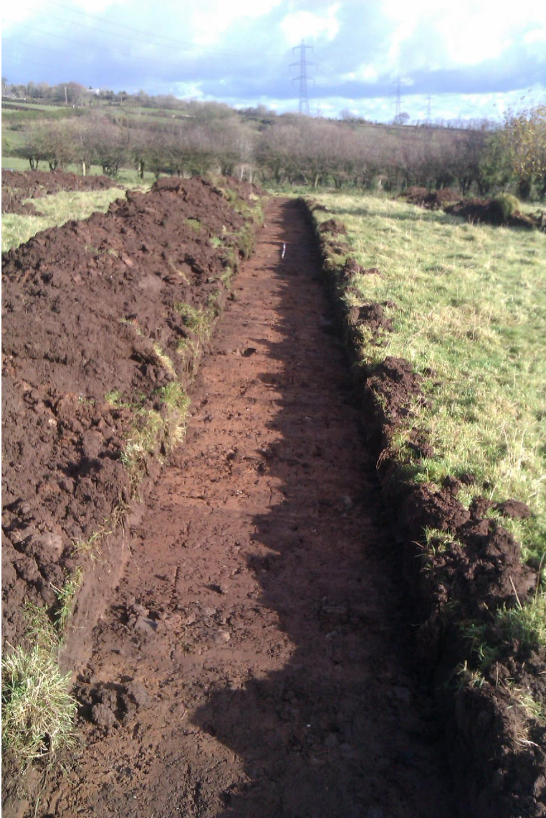
Plate 15: General view of Trench 3 following excavation to subsoil level, looking east
