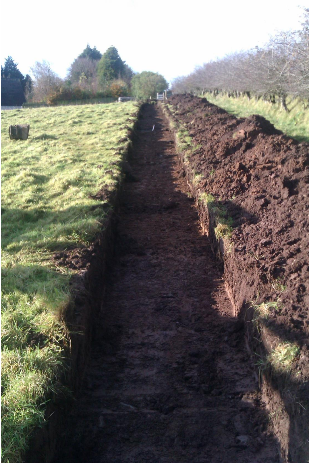
Plate 5: General view of Trench 1 following excavation to subsoil level, looking west
