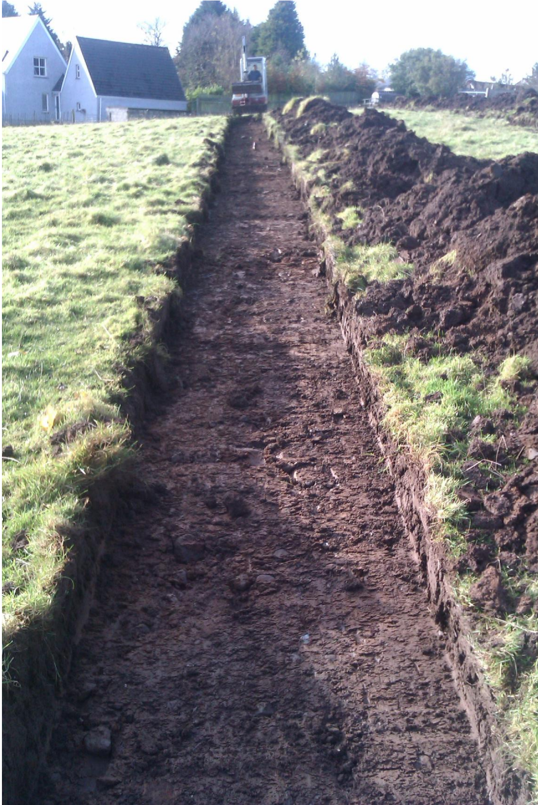
Plate 18: General view of Trench 4 following excavation to subsoil level, looking east
