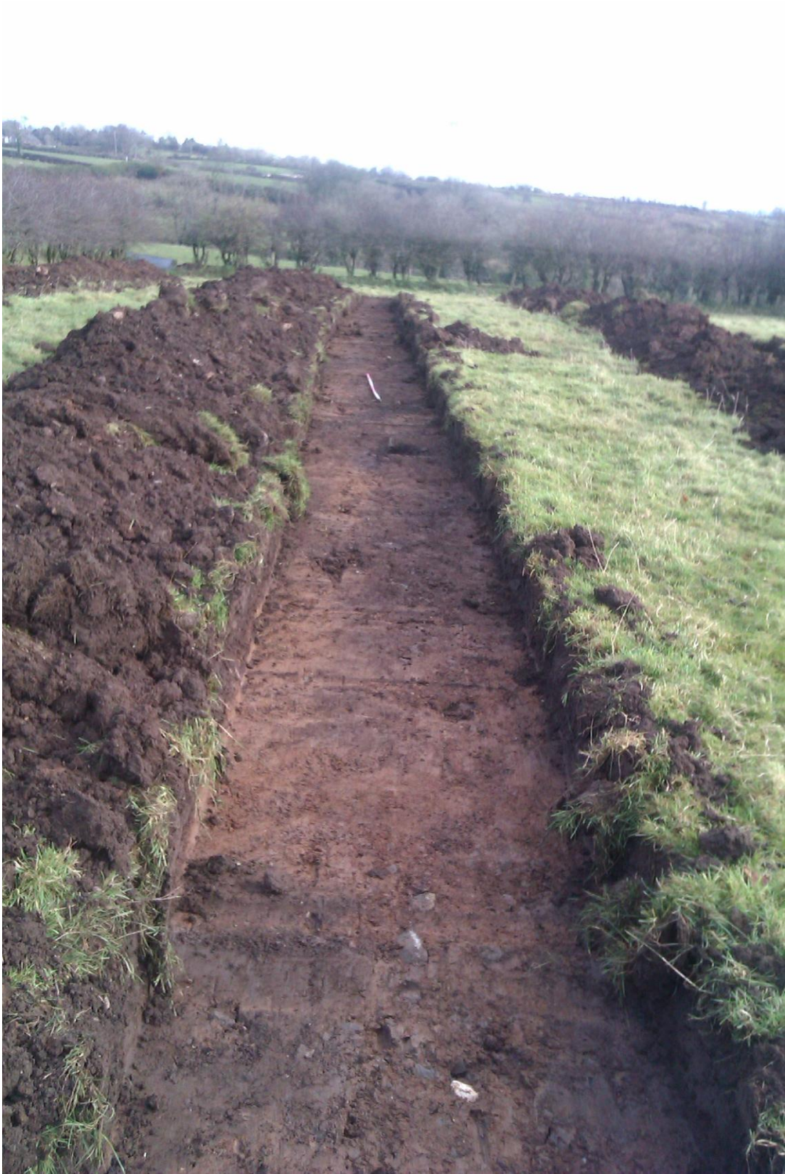
Plate 10: General view of Trench 2 following excavation to subsoil level, looking east
