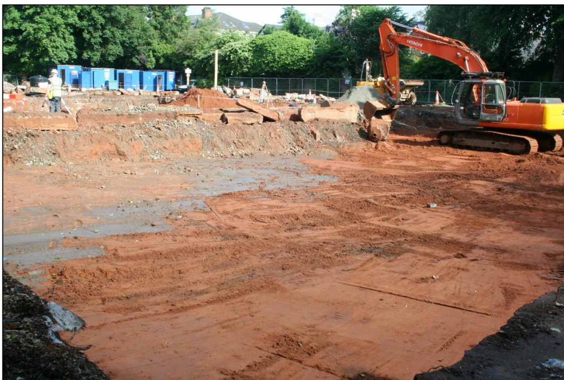
Plate 2: Levelled subsoil surface in Block A (variation in colour is due to lying water)
