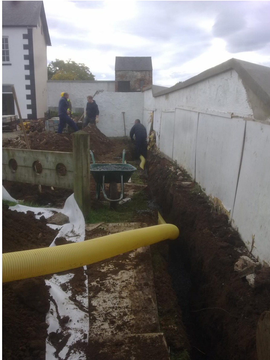
Plate 4: Excavation of Trench Two and installation of drainage pipe, looking south.
