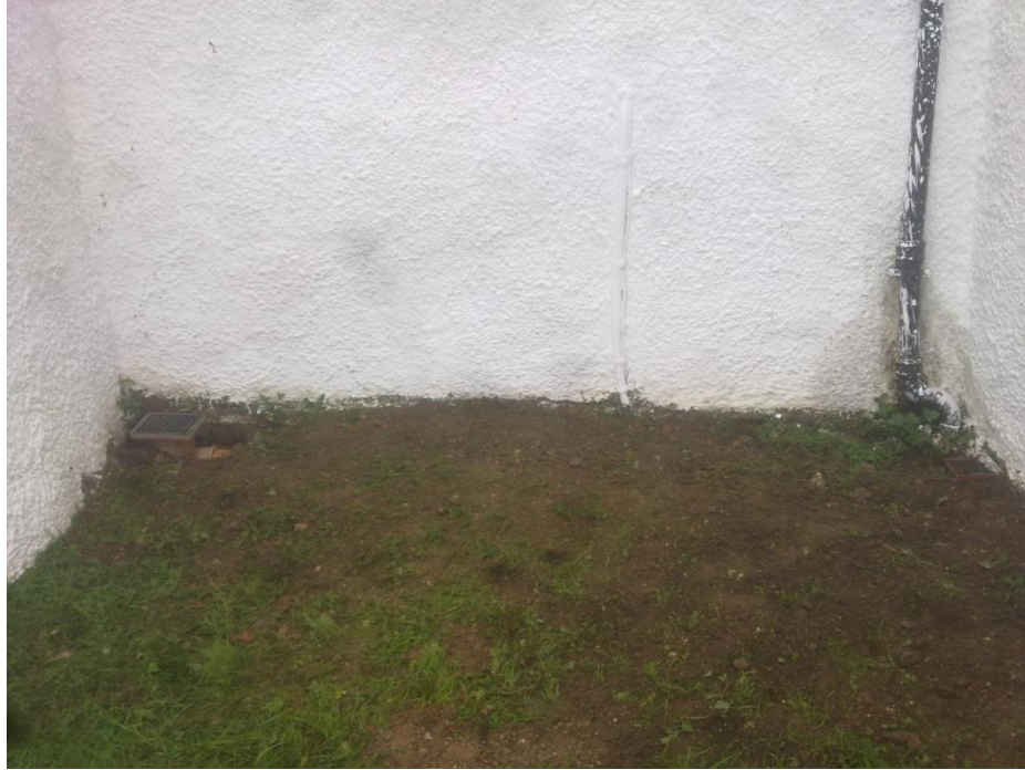
Plate 3: Trench One following backfilling, looking west.
