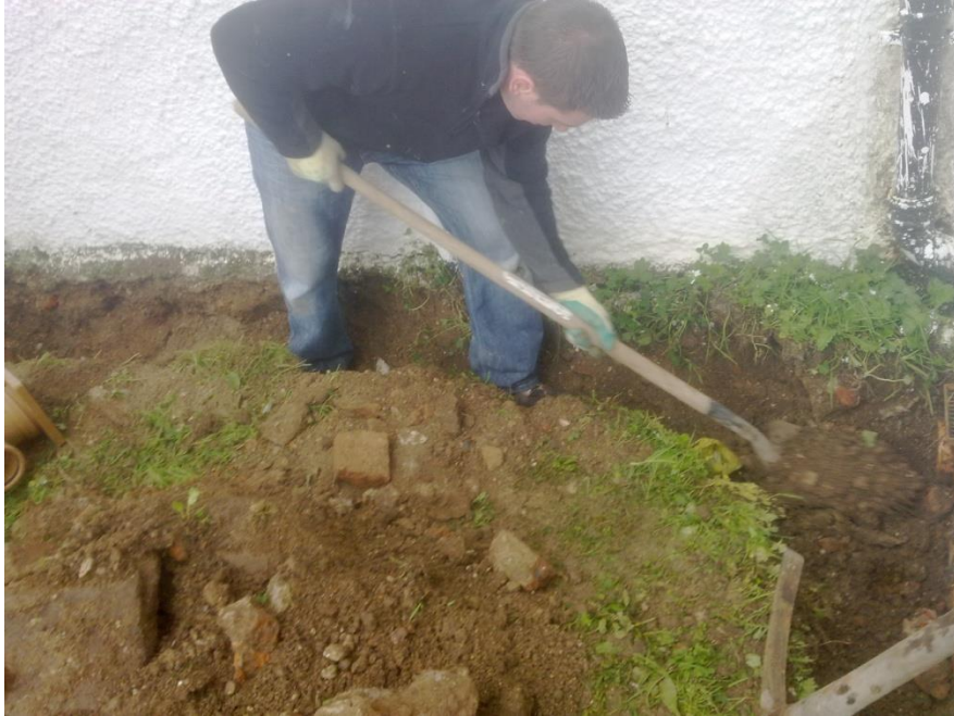
Plate 1: Manual excavation of Trench One, looking west.
