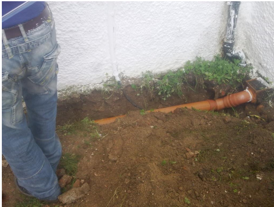
Plate 2: Installation of drainage pipe in Trench One, looking north-west.
