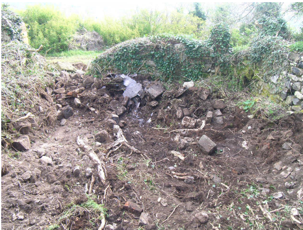
Plate 03: South-west room after removal of rubble, looking south
