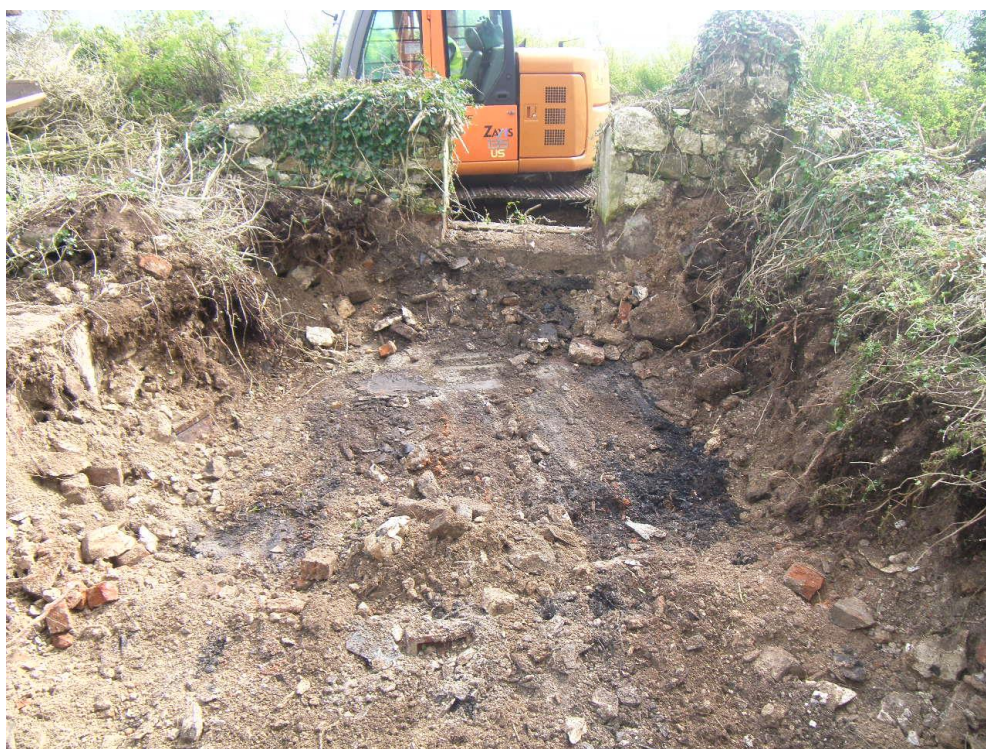
Plate 04: Centre room after removal of rubble, looking south
