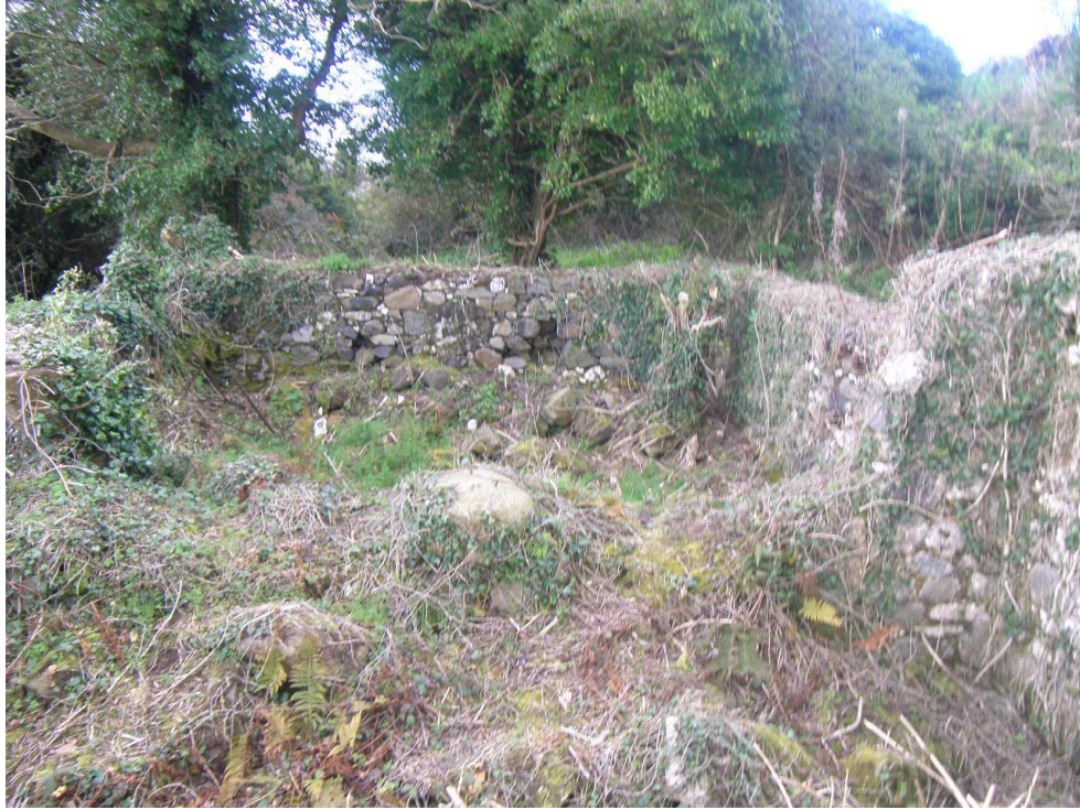
Plate 01: View of building remains before removal of rubble, looking south-west
