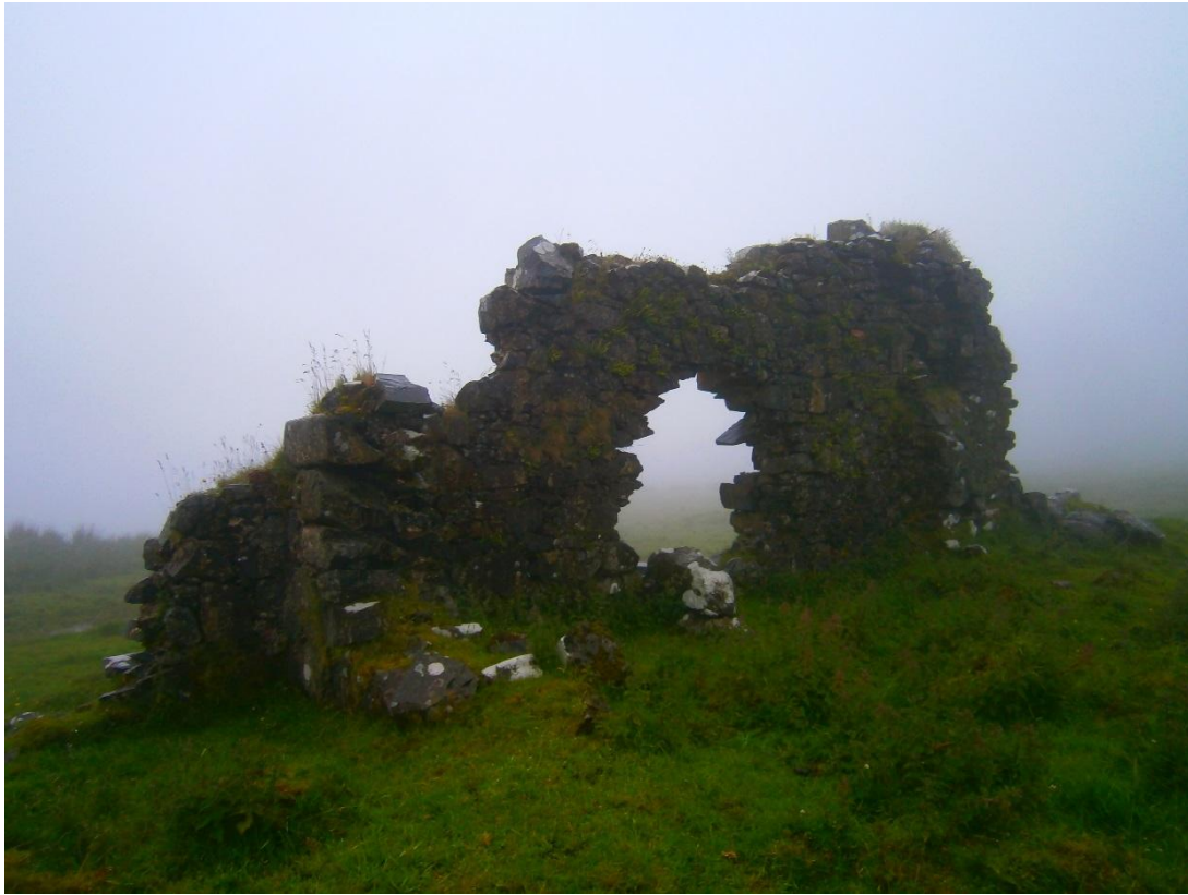
Figure 4: The northern gable of the dwelling house, 4 th July 2016
