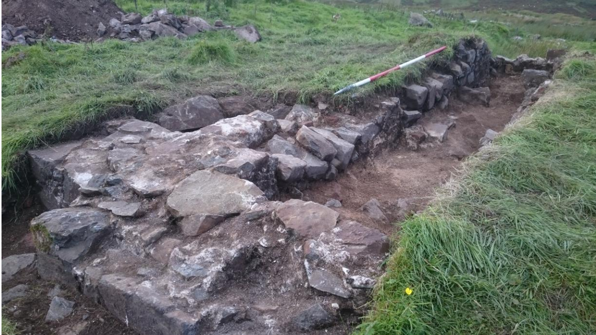
Figure 27: View of Trench Three during its excavation, showing the thick deposit of mortar (Context No. 303), looking west.
