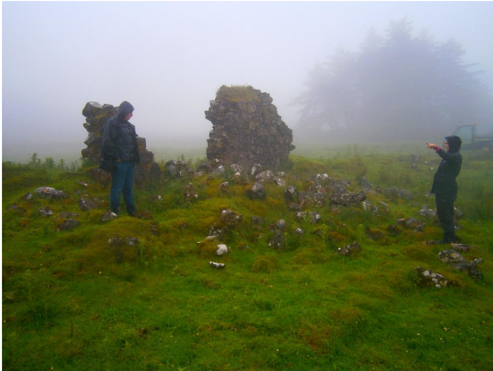
Figure 5: The remaining sections of upstanding masonry within the interior of the dwelling house, 4 th July 2016.
