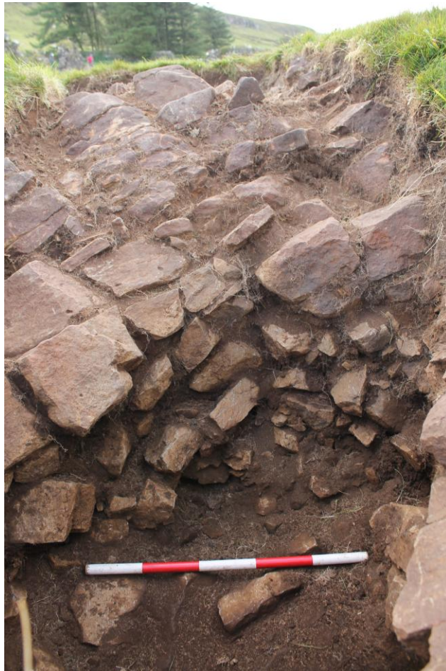
Figure 39: Detail of the structure of the kiln (Context No. 505), looking south-west (scale = 0.5m).
