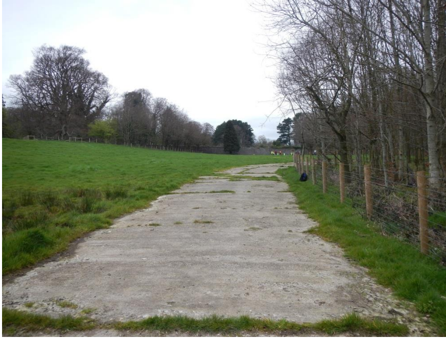
Figure 07: View of eastern access road, looking north
