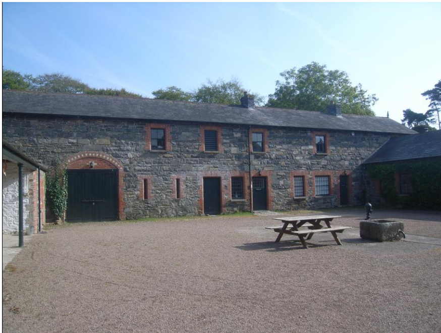
Figure 08: Stable yard with gate to threshing area
