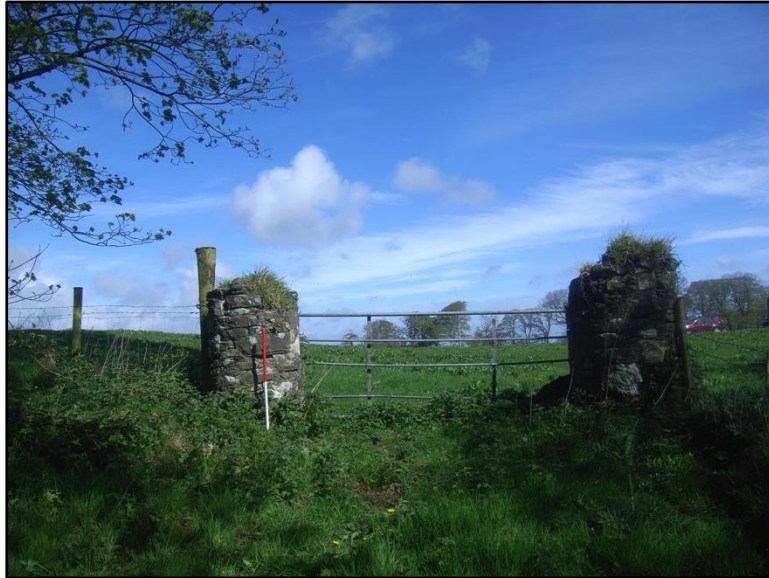
Figure 05: Two gate pillars (one with top stone missing)
