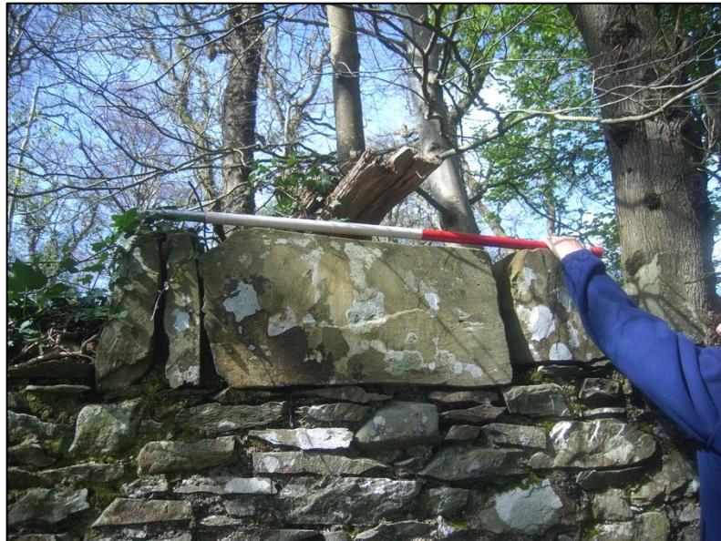
Figure 6: Large cut stone re-used in the construction of a nearby wall
