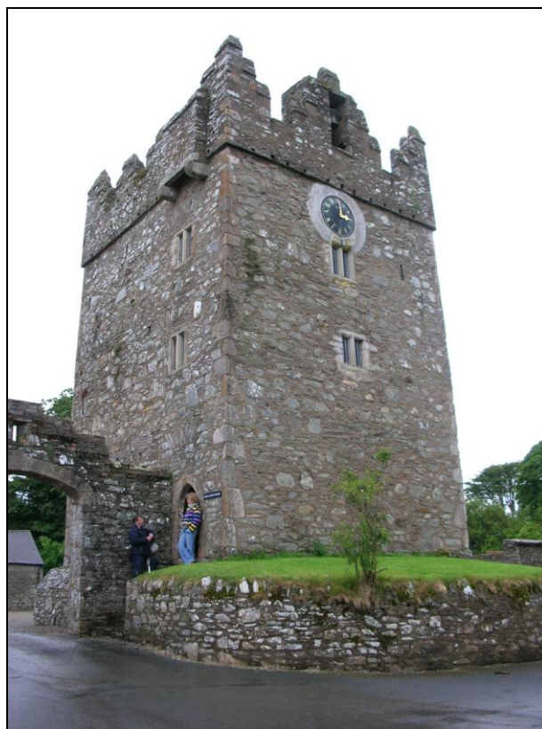
Figure 15: View of Old Castle Ward from north-east, with possible adjoining Jacobean house on left
